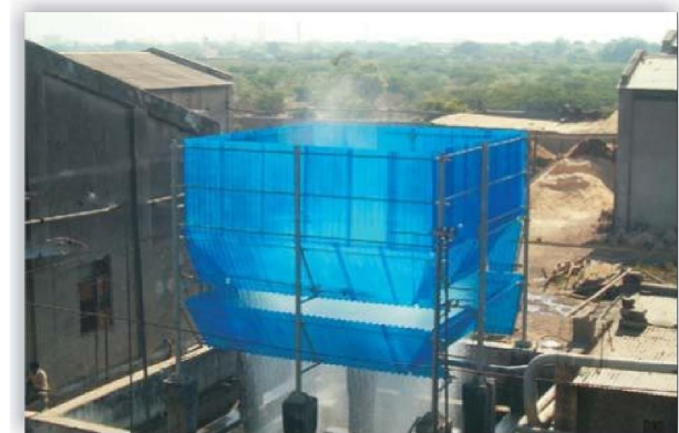
LTMCS installed on existing Cooling Tower pit
